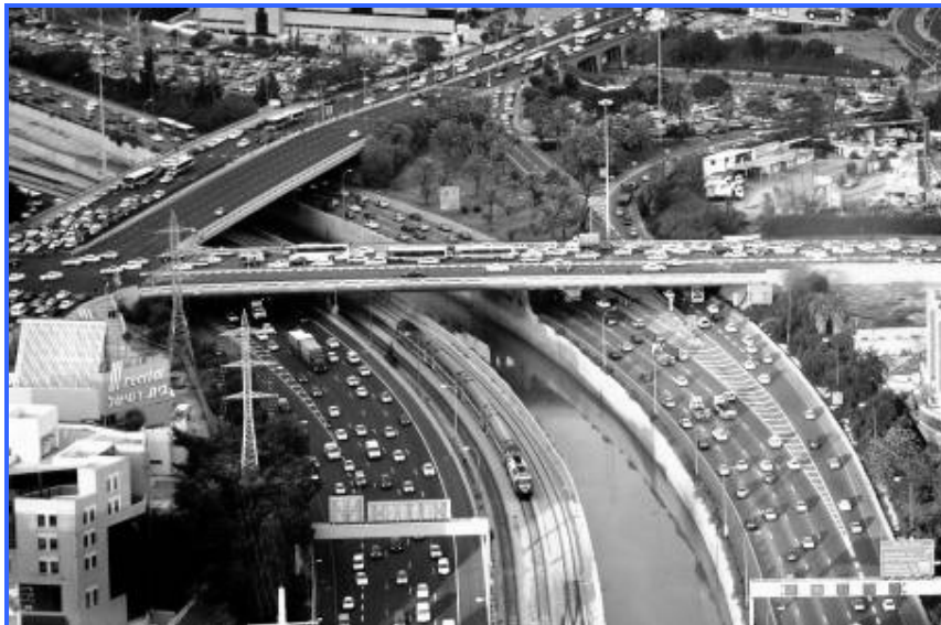
THE ISRAEL RAILWAYS ALIGNMENT AT ARLOZOROV IN CENTRAL TEL AVIV
